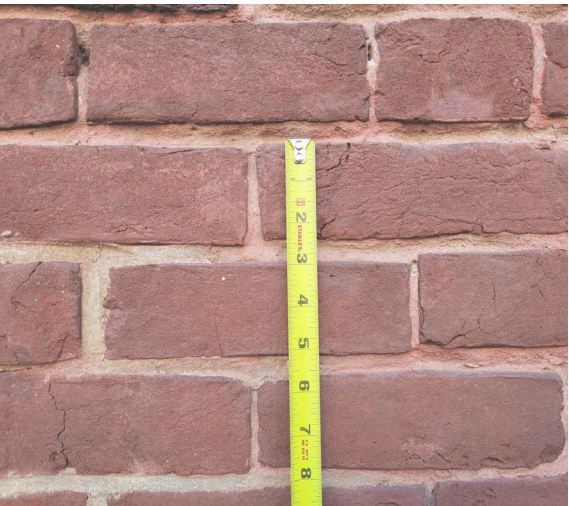
MEASUREMENT OF EXISTING BRICK ON HISTORIC WERTENBAKER HOUSE
